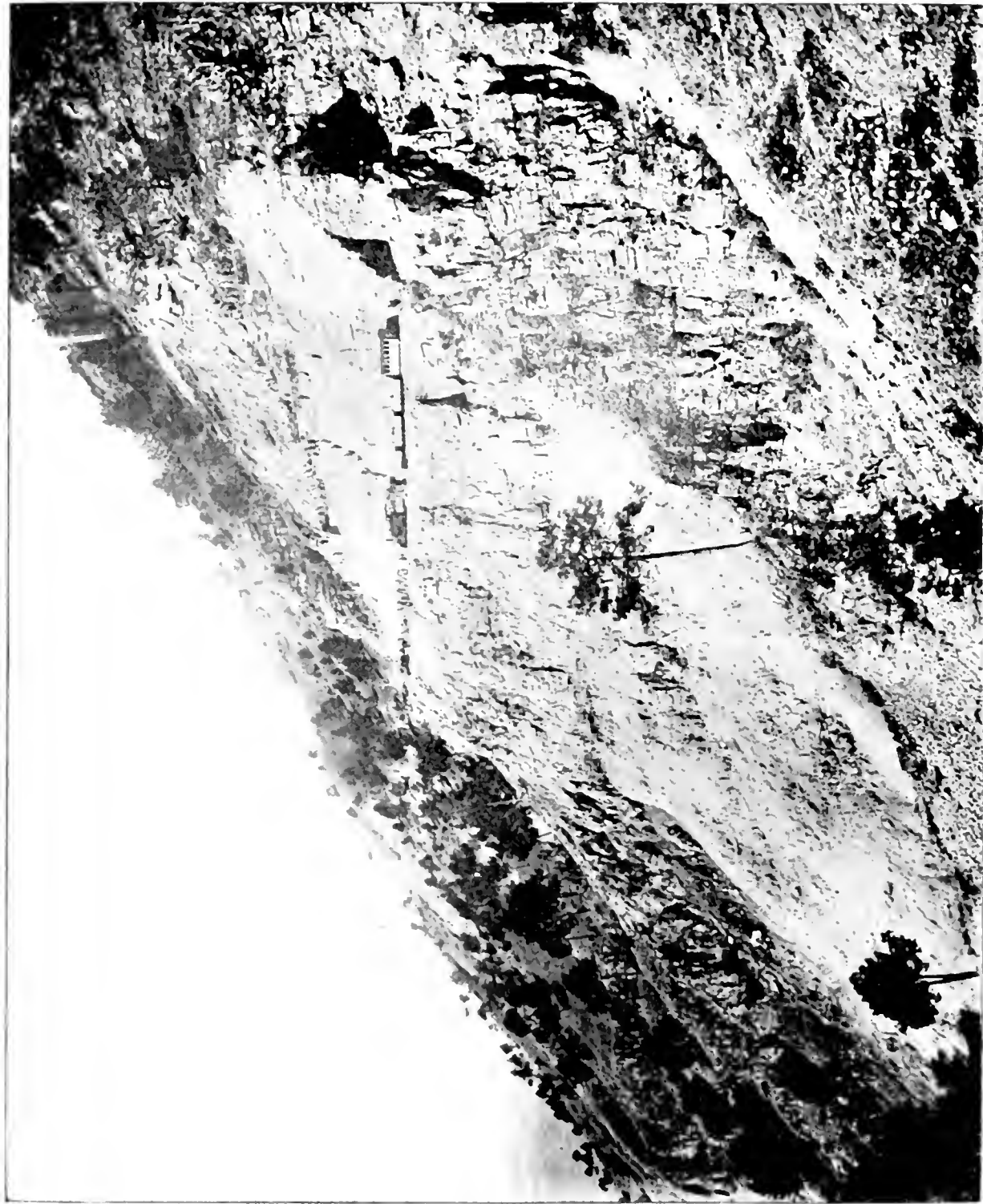
THE SIMLA KALKA RAILWAY. (A HILL SLEEP AND BREAST WALL).
